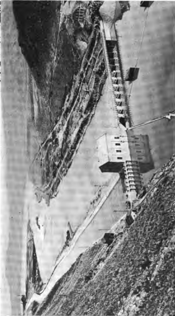
FIG. 93.—Boise Dam, Canal and Headworks, Boise Valley. Headgates in line with Dam.
